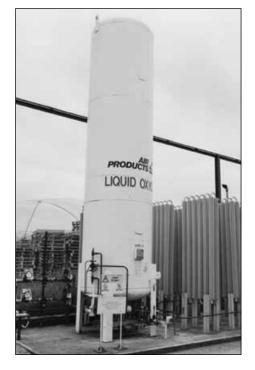
Figure 4Bulk supplystorage – liquid oxygen
