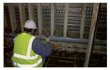
Scraping away excess material during pouring
